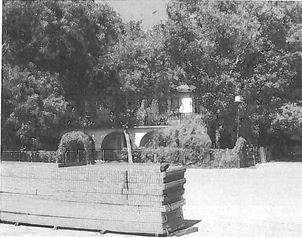
Resource # 77A, looking NE. Photo taken through gap in fencing.
