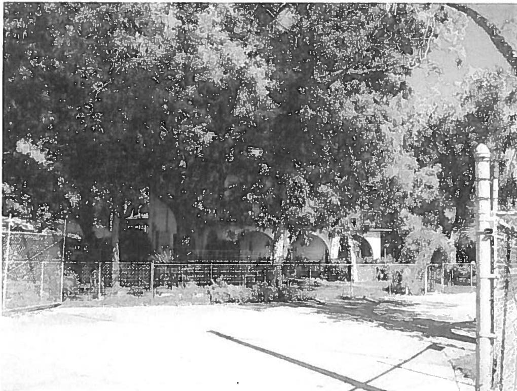
Resource # 77A, looking NE. Note the heavy vegetative screening.
