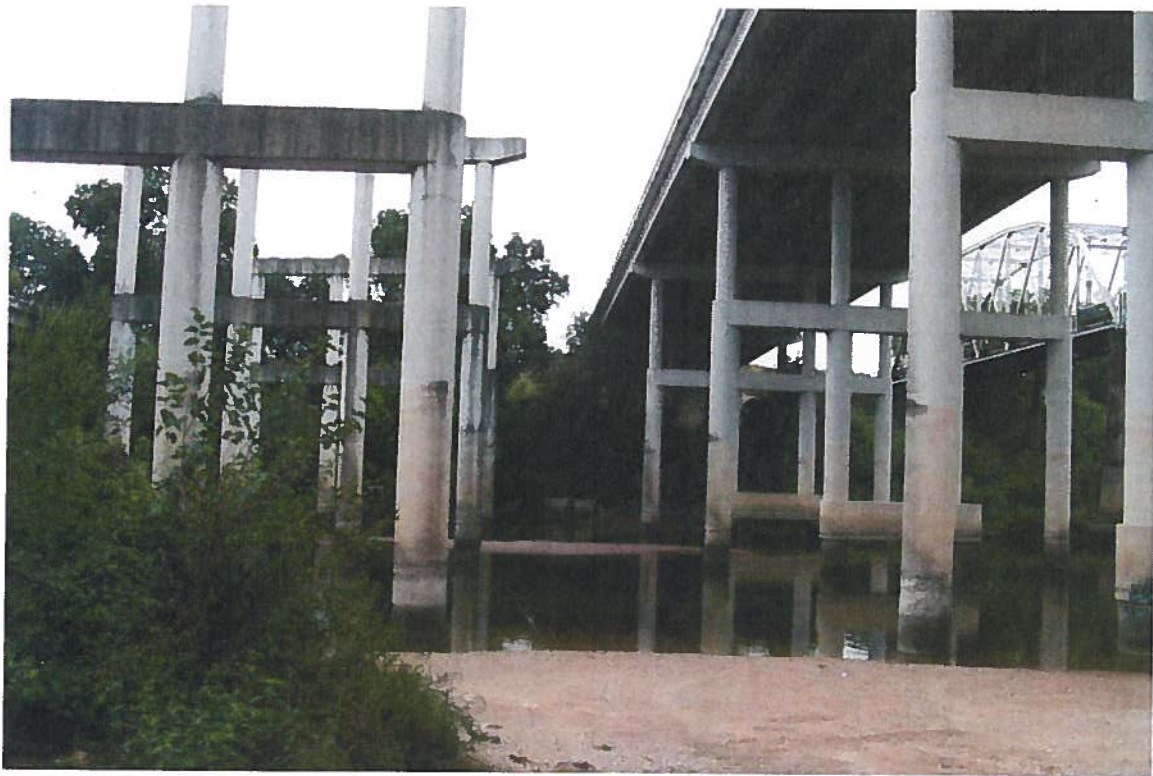
Proposed Southbound mainlane (SBML) bridge view from north to south bank. Bridge will be constructed by widening existing structures.
