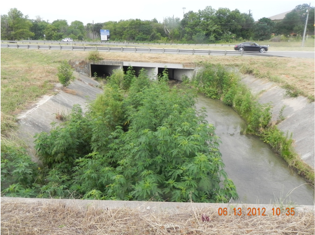
Standing east of US 183 looking west at Montopolis Tributary.
